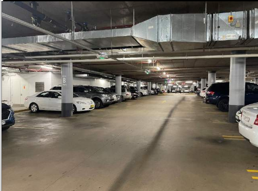
PHOTOGRAPH 3: INDICATIVE BASEMENT PHOTO
